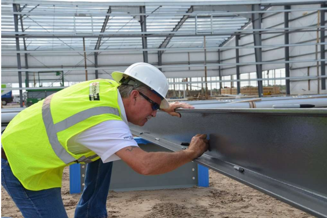
West Villages Development Director Brad Soule signs the beam.
